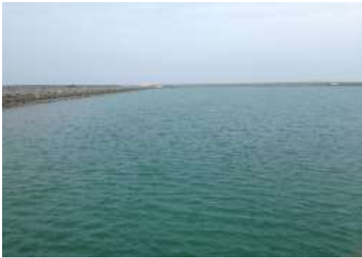
Open Intake Continuous Chlorination
